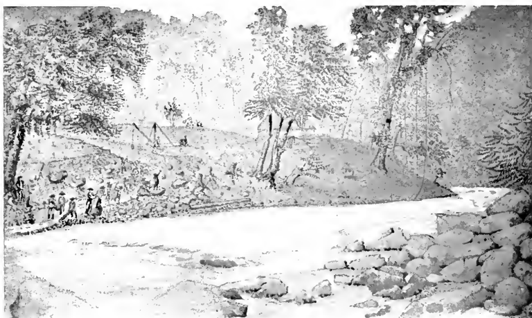
"VERANEO." CLEARING THE GROUND PREPARATORY TO BUILDING A CAISSON.
